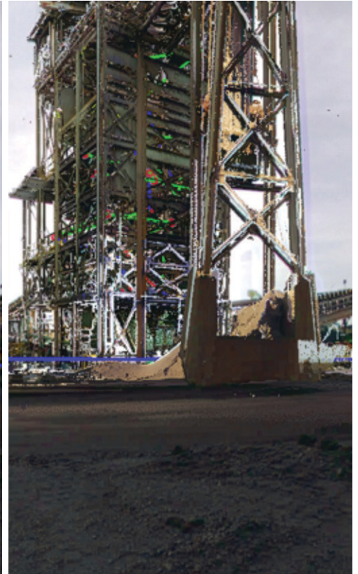
3D point cloud image
